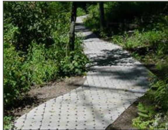
Figure 120: Permeable pavement allows water to infiltrate into the ground through the spaces between the blocks filled with fine rock. Two layers of rock below the pavers provide a strong base for the street and help the infiltration process. Geotextile fabric layers below the base rock further reduce pollutants carried into the soil as the water infiltrates
