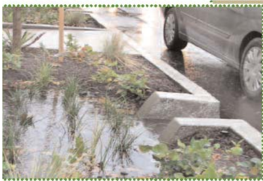
Figure 118: Biofiltration units in commercial area of Portland, Oregon.
