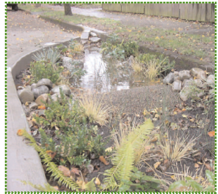
Figure 116: Biofiltration improvements in residential areas of Portland, Oregon. These filtration areas take storm water from streets through a curb cut and return the filtered water into the storm drain system.
