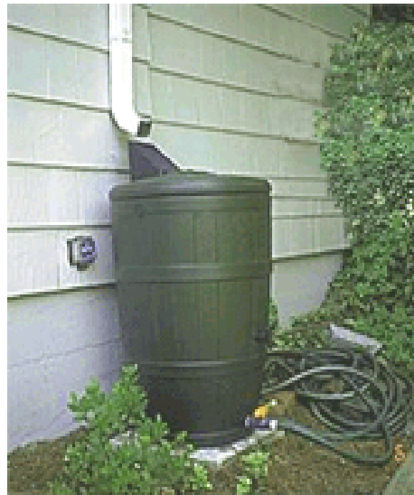
Figure 113: Rain barrels are used in many locations to collect runoff from roof areas for use in garden watering.
