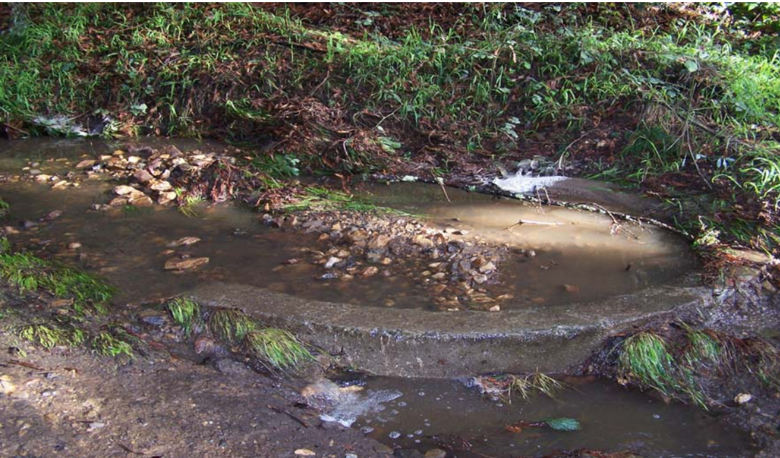
Figure 59: Top: Fern Ravine Creek, part of PSC2, in Joaquin Miller Park after the Jan 1, 2006 flood where the creek flowed out of its concrete channel and overland. Bottom: Filled-in culvert drop inlet.
