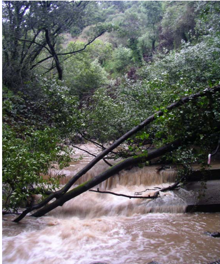
Figure 65: Grade control structures in SC1 during the Jan.1 2006 flood.
