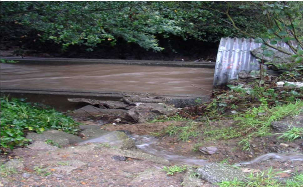
Figure 72: Top: Sausal Creek in downstream area of Dimond Park where private residences border the creek (SC3). Failed gabions (rock-filled baskets) remain from prior bank stabilization project. Bottom: Large culvert carries Sausal Creek under meadow.
