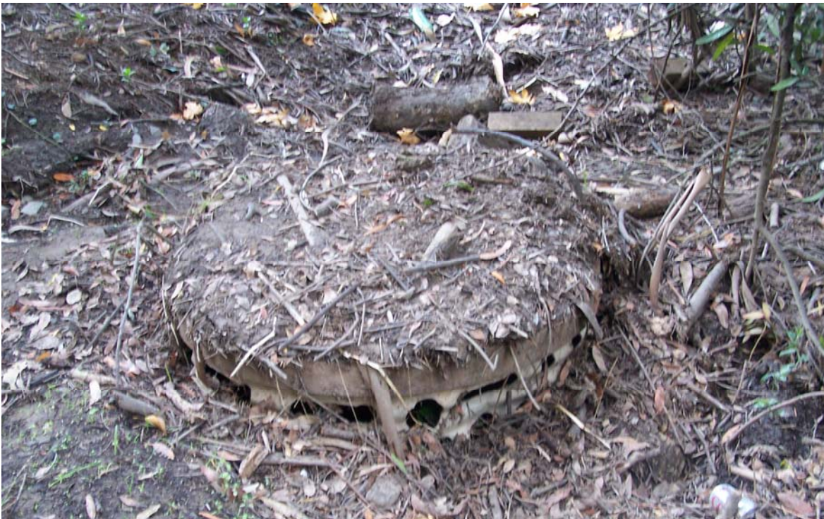
Figure 57: Top: Tributary to Cobble Dick Creek along Larry Lane (CC1) flows into a sediment basin. Bottom: Lack of maintenance of basin shows in this buried and largely nonfunctional standpipe.
