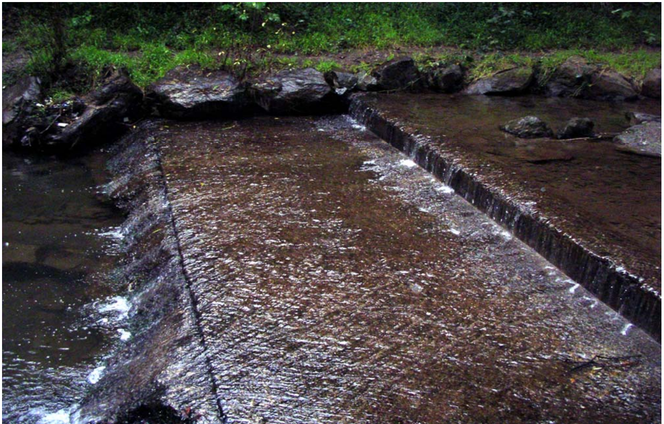
Figure 64: These photos are examples of the drop structures in Sausal Creek (SC1) in Dimond Canyon.
